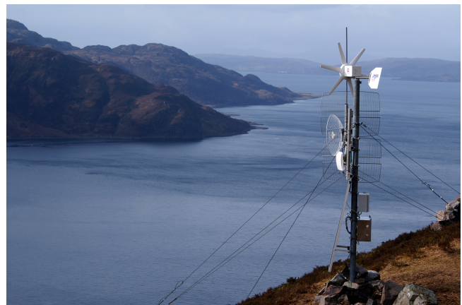
Figure 2: Self-powered mast on Beinn Sgritheall (node B in Figure 1).
